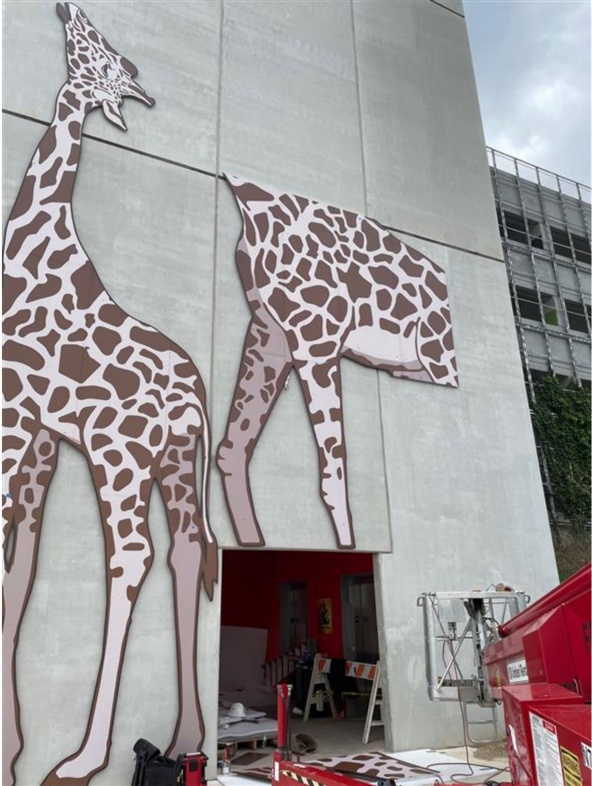
Brackenridge Parking Garage (in progress)
