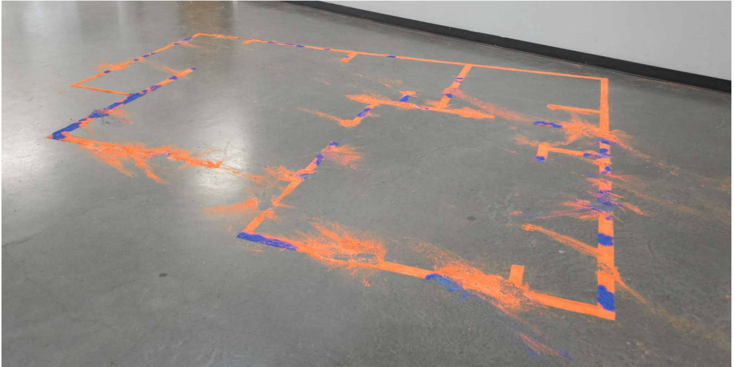
Floor, Floor Plans II , Day 5 (Before Repairs)
