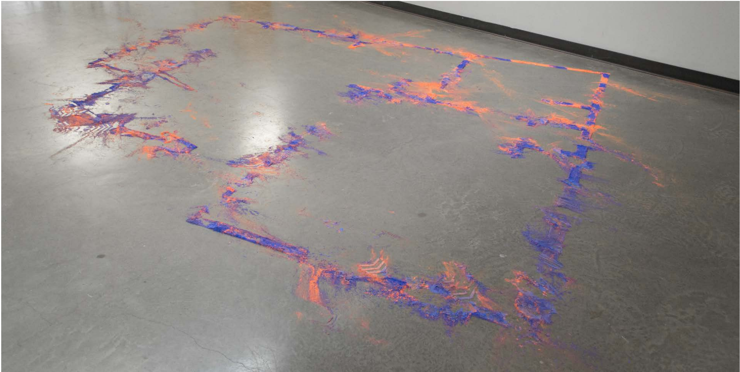
Floor, Floor Plans II , Day 6 (Before Repairs)
