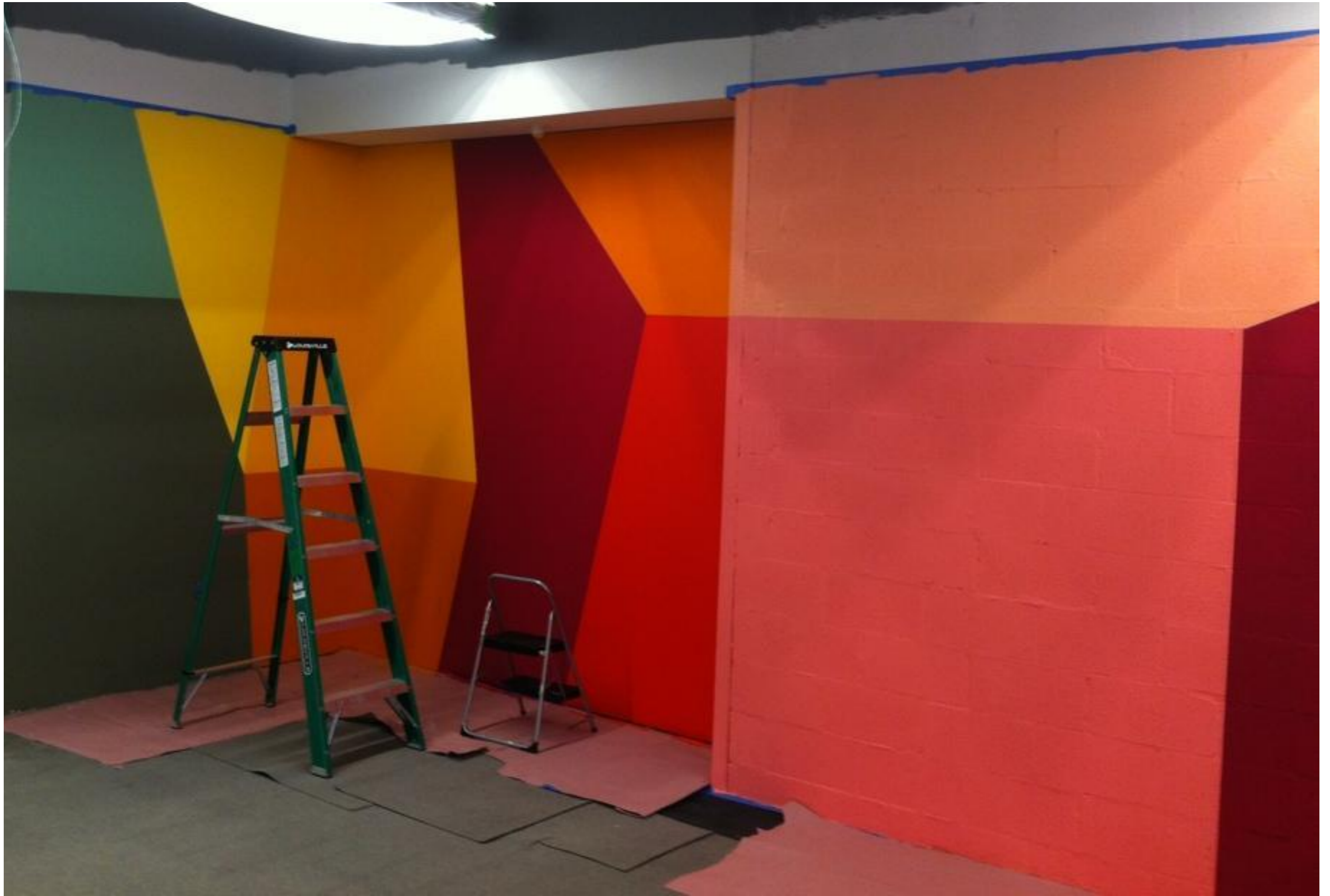
Pulse Fitness (Progress Image), Greenway Plaza, Houston, Texas, 2016
