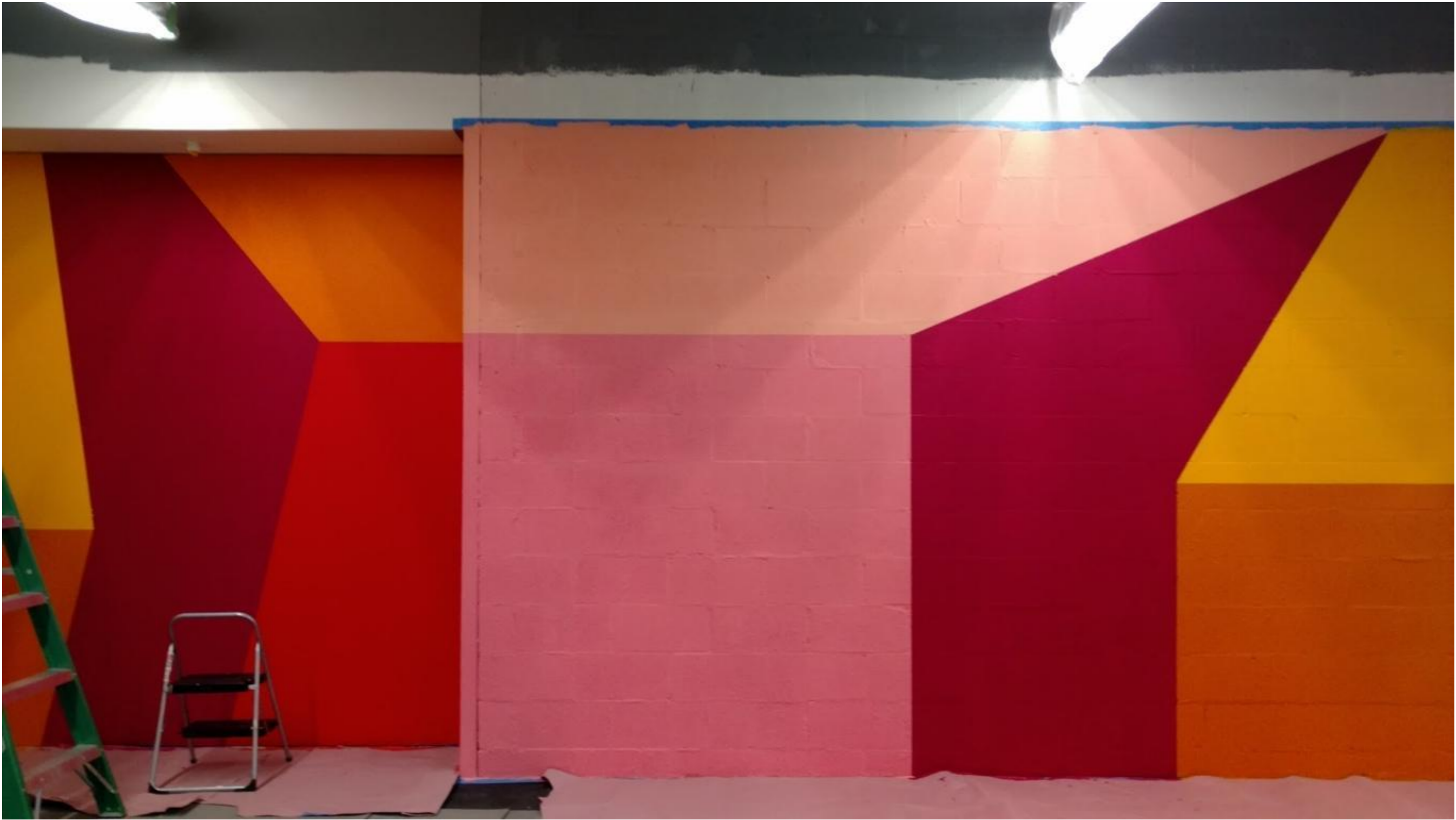
Pulse Fitness (Progress Image), Greenway Plaza, Houston, Texas, 2016
